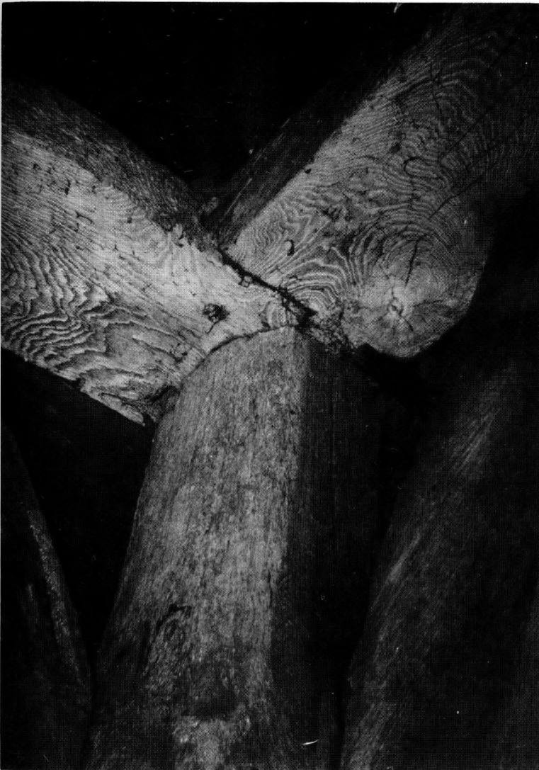
Fig. 36 Stock belfry, Essex, showing a late top- plate before the mitred joint
